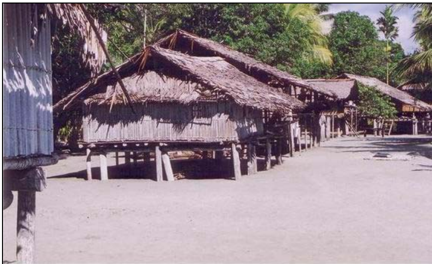
The Maisin village of Airara with sago-leaf roof topped houses.
